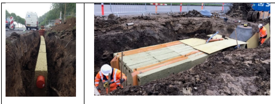
Left: Construction of a pilot-scale filter at Strandvejen
