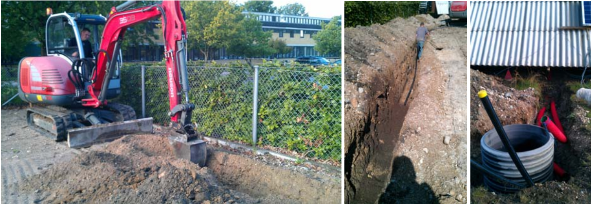
Figure 2. Pictures taken during the construction of the ground source heat exchanger.
