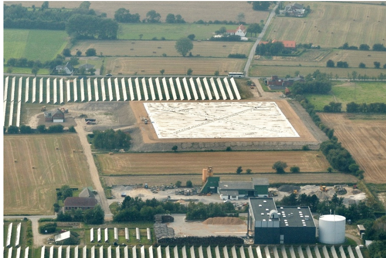
Fig. 1: Bird view of the water pit heat storage in Marstal Solar heating plant
