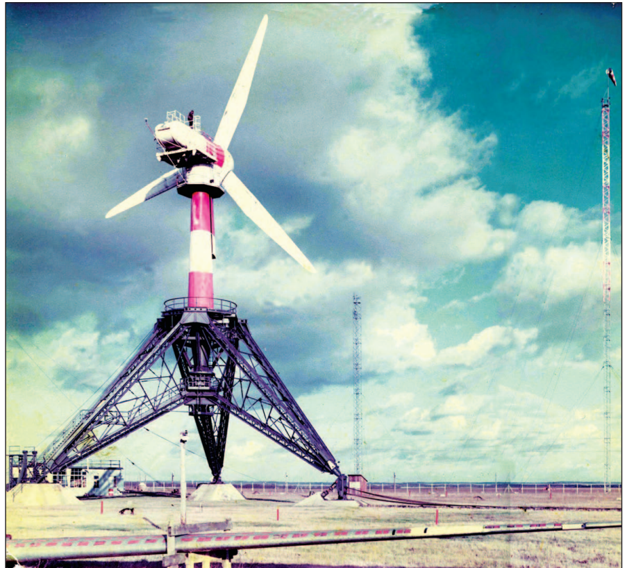
FIGURE 6 – The experimental 800-kVA BEST-Romani aerogenerator (wind turbine) put into operation in Nogent-le-Roi, France, in 1955. (Photo courtesy of Jean-Luc Cavey.)
