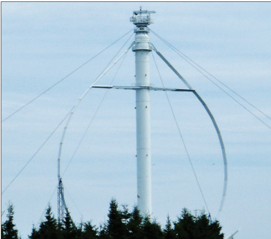
FIGURE 8 – The Éole, a 4-MW 110-m Darrieus's vertical-axis wind turbine installed at Cap Chat, Gaspésie, Quebec, in 1987 is still the largest in the world. A fault in the base bearing put it permanently out of service in 1993.
