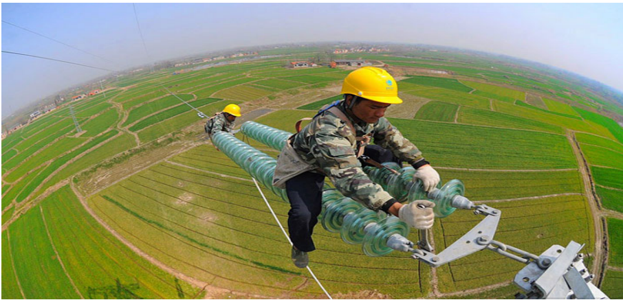
Figura 12. High voltage tower inspection.
