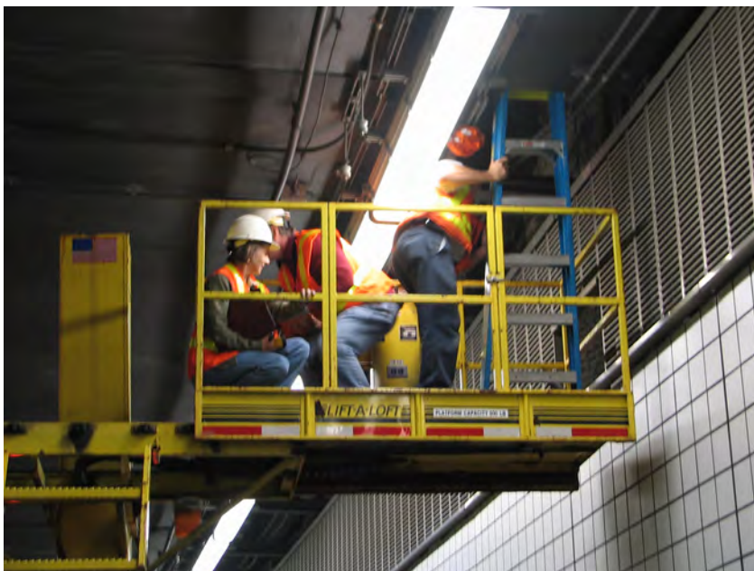
Figure 2.5 Equipment and location of access for tunnel inspection
