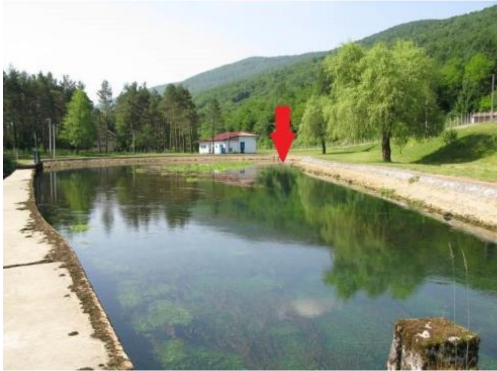
Figure 3: Zagorska Mrežnica spring cave after the construction of the pumping station.
