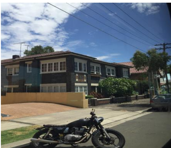
The pedestrian walkway is well maintained and levelled across all houses in the neighbourhood
