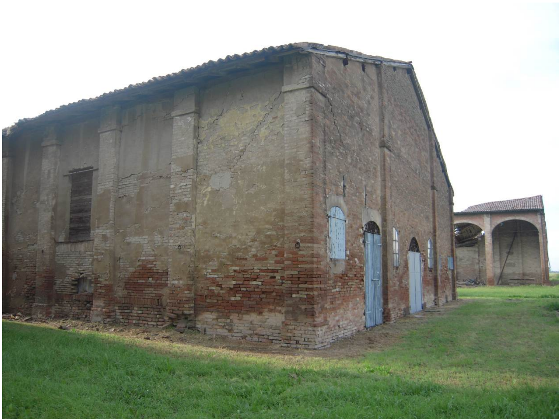
Fig. 7. Damage at corners: a) Unreinforced masonry building in Los Angeles 1994 Northridge Earthquake (photo by D.P. Abrams); b) Rural building after the Emilia 2012 earthquakes (Sorrentino et al., 2014).
