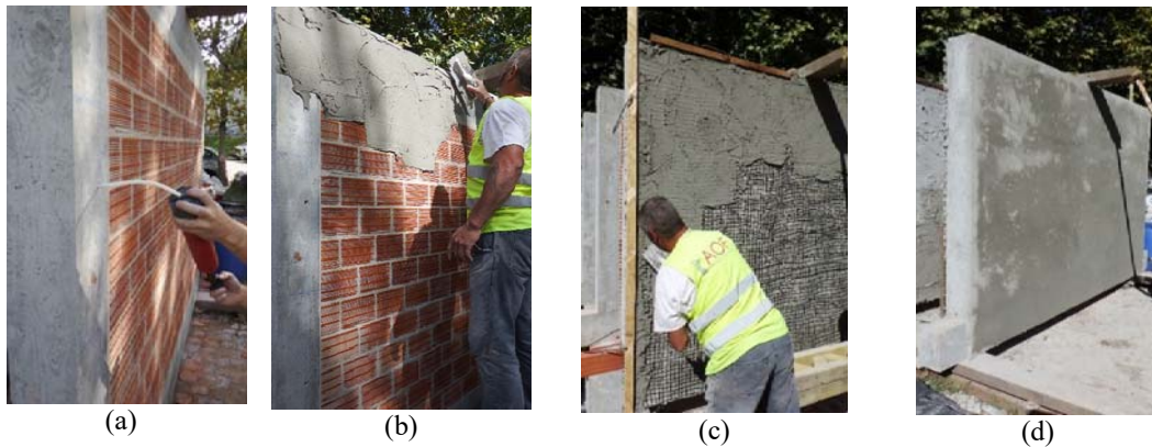
Figure 5 Application of the reinforced rendering; (a) drilling the pilot holes (b) applying the first layer of mortar (c) positioning of the textile mesh and application of the second layer of mortar; (d) final aspect after rendering
