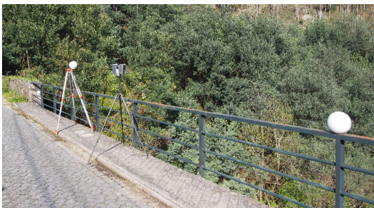
Figure 3. Recording system during the geometrical characterization of the bridge
