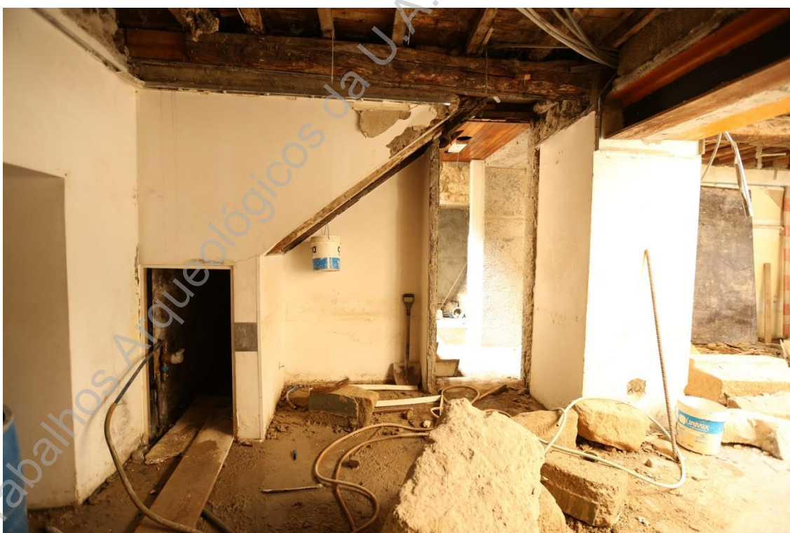
Foto 28: (UAUM-IMG_6155) Pormenor da parede interior do piso 0 (UE013, UE016, UE012) O-E.
