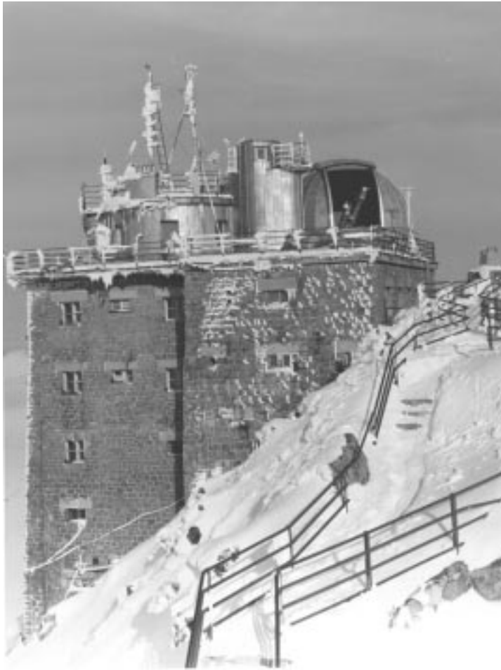
Fig. 1. – Solar corona observatory of the Astronomical Institute of the Slovak Academy of Sciences (Mt. Lomnický Štít, 2632 m a.s.l.; inside the cupola the double solar coronagraph: D = 20 cm, f = 400 cm).
