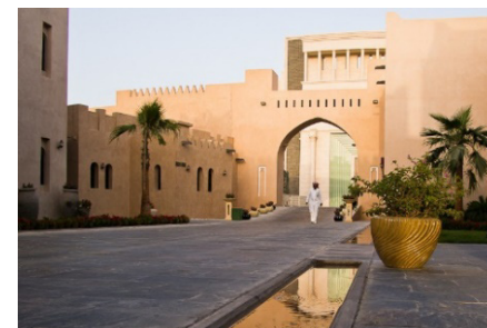
Figure 19–20. The Katara Amphitheater, exterior
