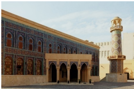
Figure 16. Mosque in Katara Cultural Village, Doha, Qatar
