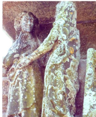
Figure 1.5 - Colonization of a statue with lichen, figures from the Calvary near Concarneau in Brittany [26].
