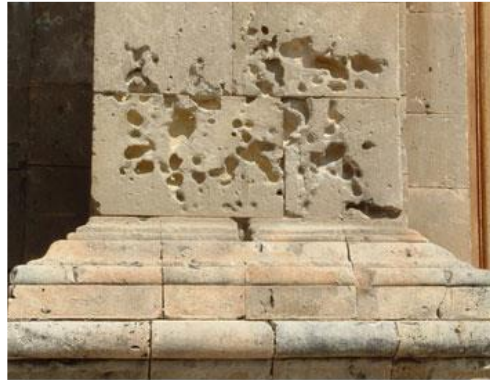
Figure 1.4 - Examples of alveolization on Noto stone (church of S. Francesco) [36].
