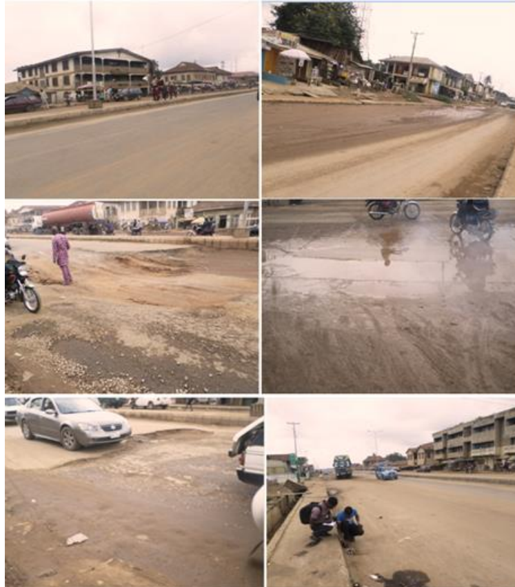
Plate 2: Snapshot of some stable and deteriorated portion of the study area.
