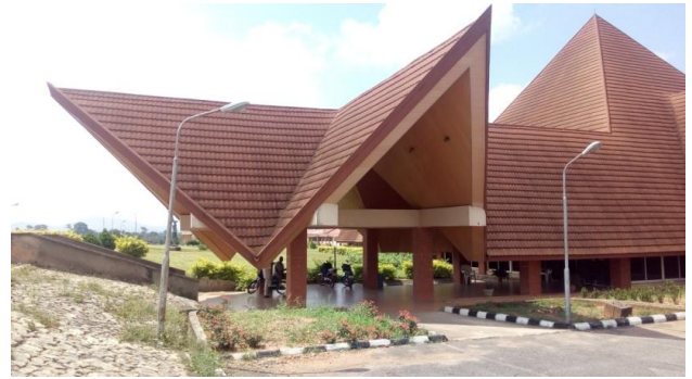
Figure 2: Access from the Car Park
