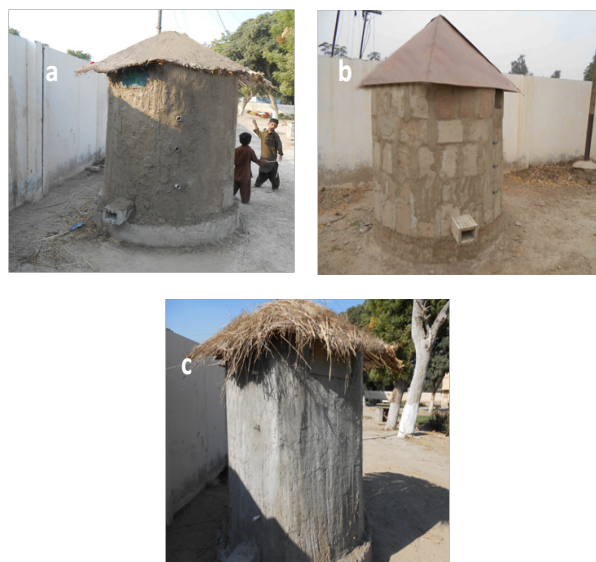
Figure 2. Three different types of designed grain storage bins used in the study (a-Straw-clay bin, b-Concrete block bin, c-Ferrocement bin)
