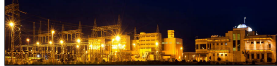
Figure 12: Night view towards Rusheder Power Plant
