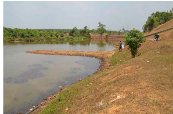
Figure 3: Visual of water condition at the site
