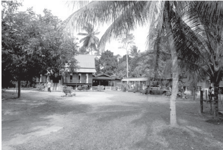
Figure 7: Original compound view without renovation showing a classic open lawn concept for Malay compound (Source: Author)
