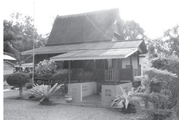
Figure 8: Original compound view with renovation showing limitation of space, and usage of petite, low maintenance decorative plants (Source: Author)
