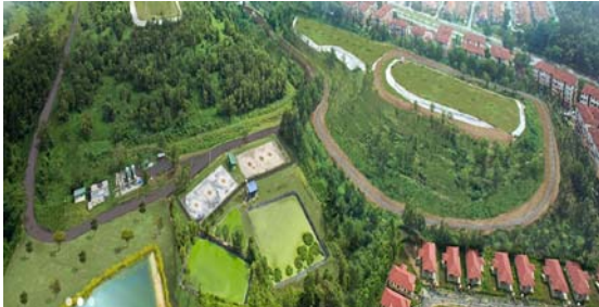
Figure 1: Existing Site Conditions of Air Hitam Puchong landfill
