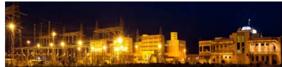
Figure 12: Night view towards Rusheder Power Plant
