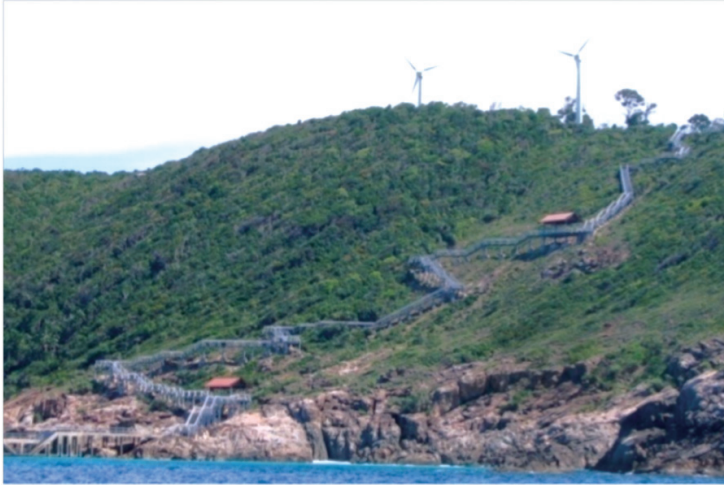
Figure 54 200 kW wind power plant in Perhentian Island in Terengganu
