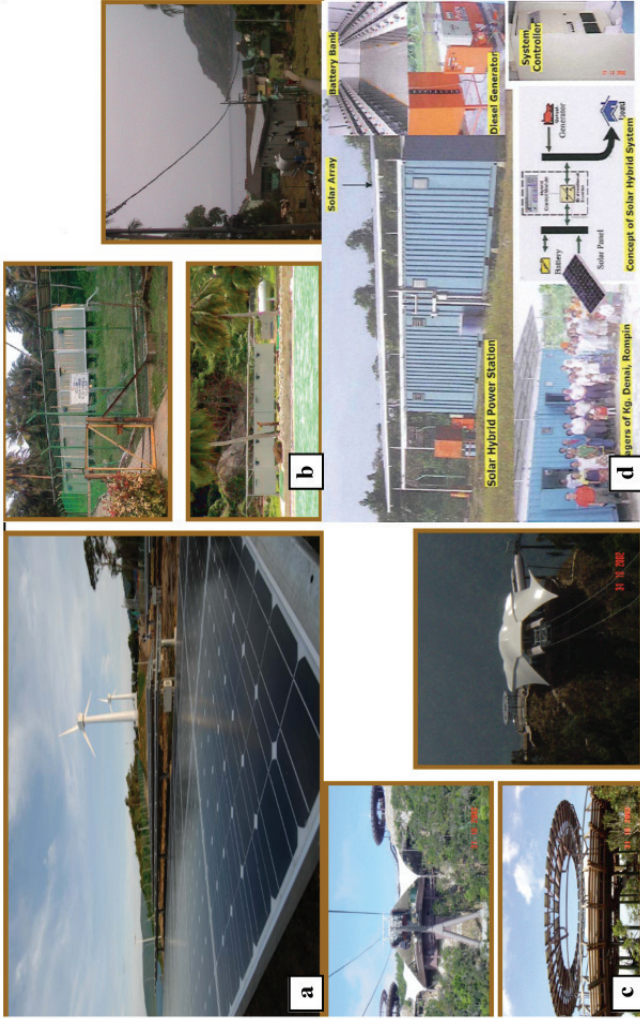
Figure 49 Solar hybrid Projects by TNB-ES in Peninsular Malaysia. (a)- Wind/Solar Hybrid in Pulau Perhentian, Terengganu (Solar - 620 kW and Wind - 200 kW); (b) - Solar Hybrid Stations off Mersing, Johore (10 kW & 15 kW); (c) - Langkawi Cable Car, Langkawi (8 kW); (d) - Kampung Denai, Rompin, Pahang (10 kW)
