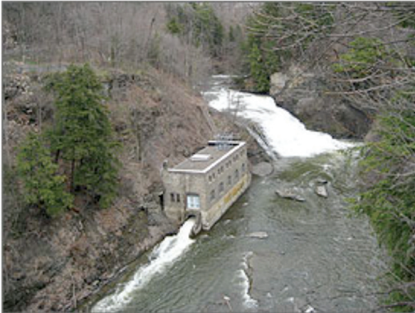
Figure 28 Cornell University leverages hydropower for electricity production through run-of-the-river facility located on Fall Creek in Ithaca, New York
