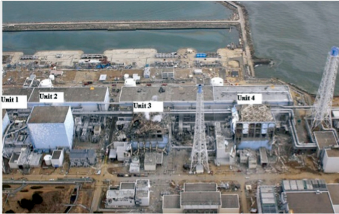
Figure 47 Explosion at Fukushima Daiichi NPP of 4 units, Japan was hit by devastating earthquake, on 12 Mar 2011 at 0630 GMT [source: BBC online, 13 Mar 2011].
