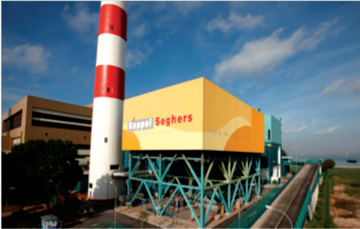
Figure 35 First WTE plant is Singapore under Public-Private Partnership initiative
