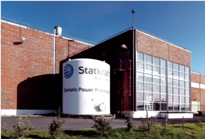
Figure 30 World's first osmotic power plant – Norway opened on 24 Nov 2009. Statkraft hopes to go all out commercially by the year 2015
