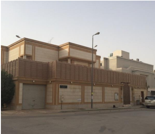
Plastic/steel shutters used for privacy (Front side)
