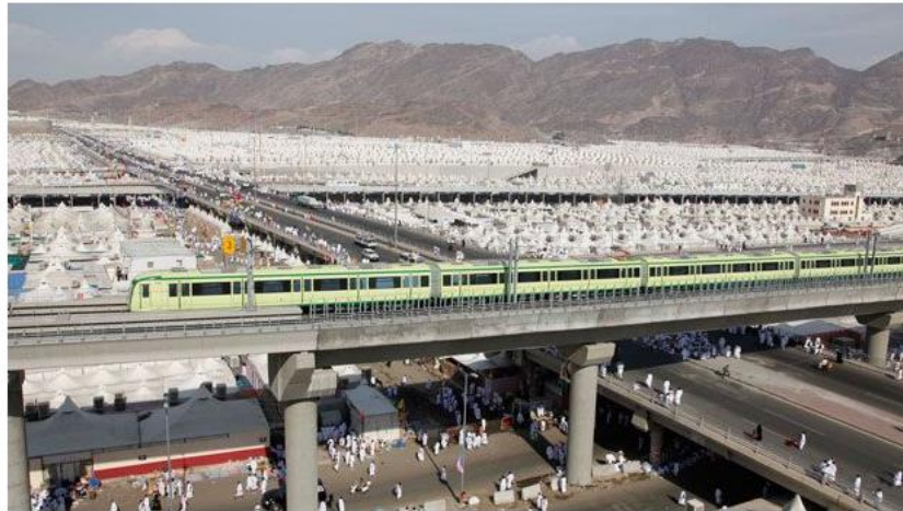
Figure B-2: Mashaier Metro project in Makkah.
