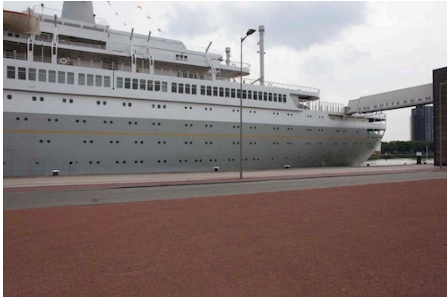
42. Exterior of the SS Rotterdam
