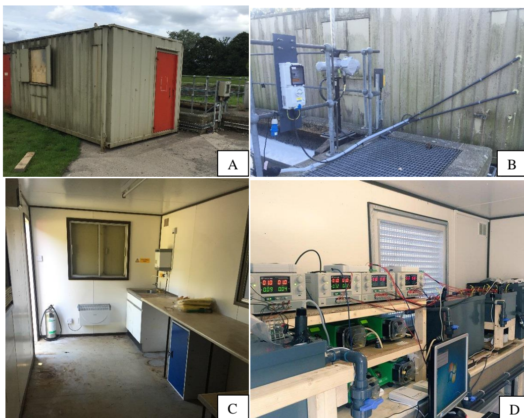
Figure 4.1 Photographs of the modified shipping container at Chester le Street STW. Modifications were made to the outside (A-B) and inside (C) of the container for it to house three MEC pilots of increasing scale (D).
