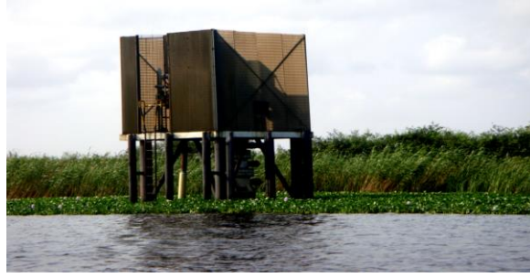
Figure 6.21: Abandoned Oil Infrastructure in Ojumole Source: Fieldwork (August 2013).
