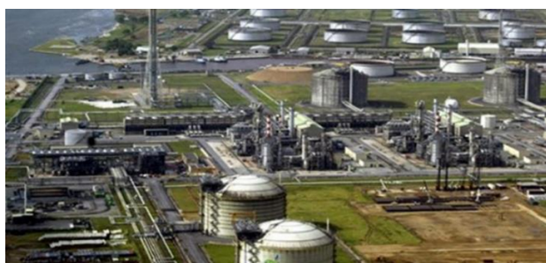
Figure 5.12: Some Oil Infrastructures in the NDR Source: NEITI (2011).
