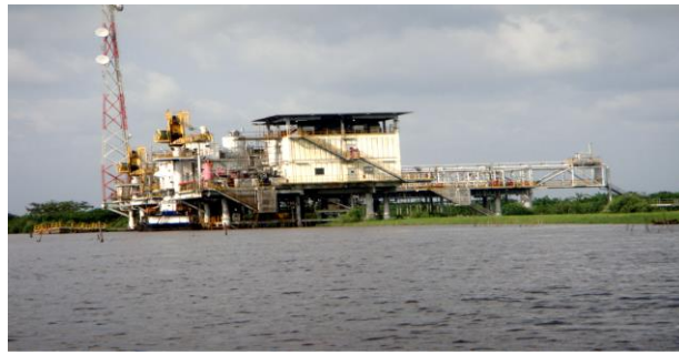
Figure 6.1: Opuekeba Oil Platform, Ondo State Source: Fieldwork (2013).
