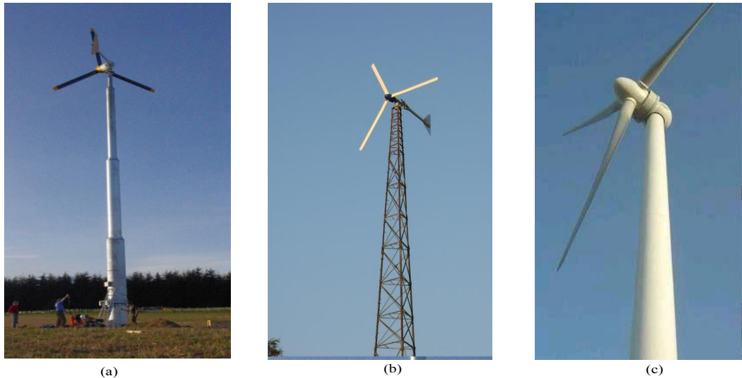
Figure 1.5: Types of tower used in wind conversion system: (a) monopole tower; (b) lattice tower; (c) tube tower [7].
