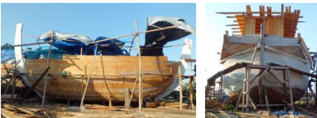
Figure 8.9 The shape of the hull on an "Ijon-ijon" in Brondong (Photo by the Author)
