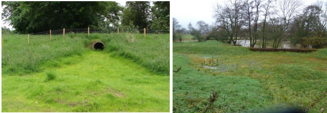
Figure 5-27 Little Ayton offline storage pond and oxbow feature; a. concrete inlet pipe to the offline storage pond; b. view of offline storage pond and oxbow in the background
