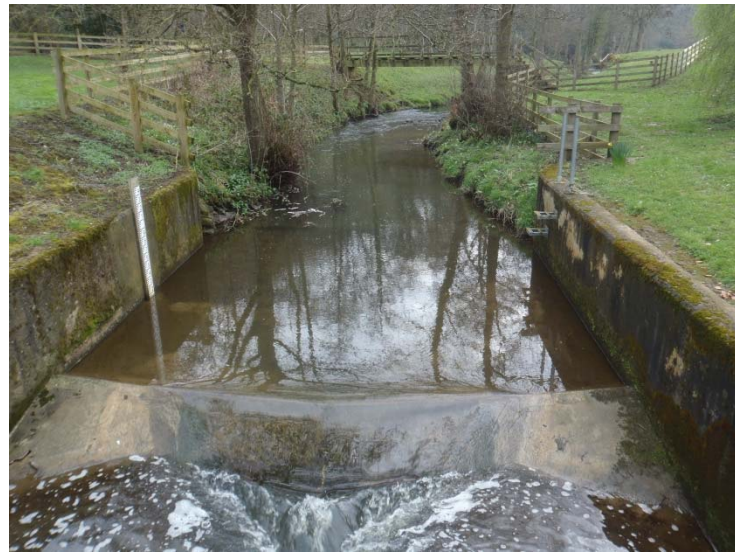
Figure 3-5 Weir at EA Easby level monitoring location
