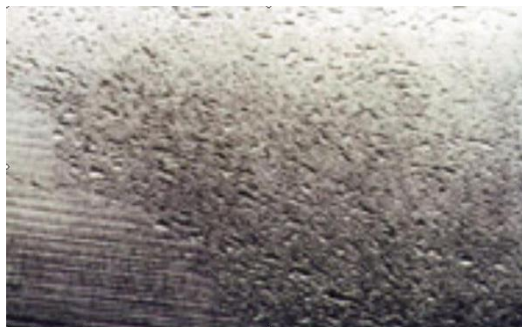
Figure 3. Micropitting damage on gear tooth surface ( www.xtek.com ).
