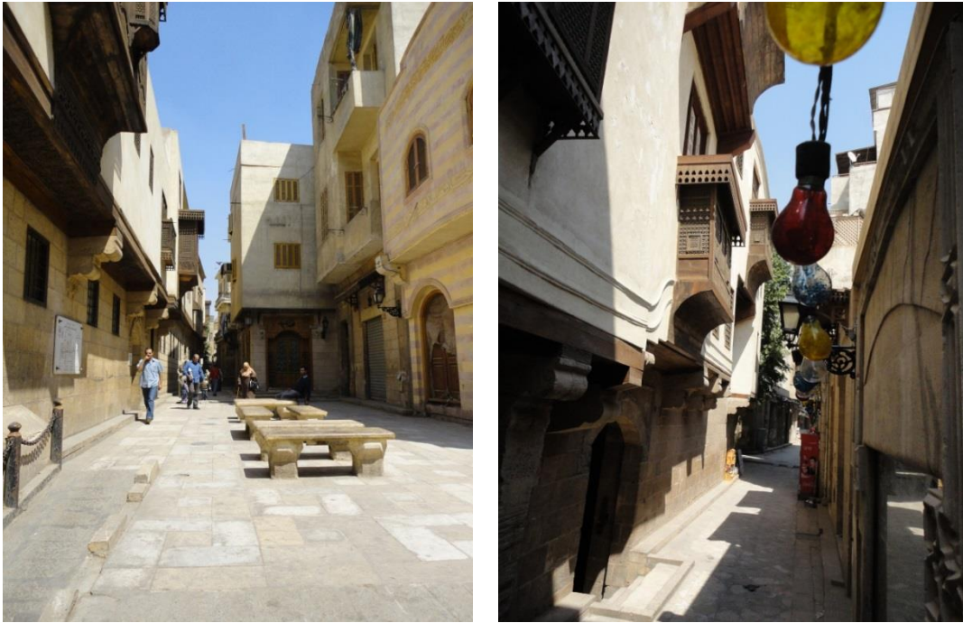
Figure 0-19A Al-Darb Al-Asfar Alley after restoration
