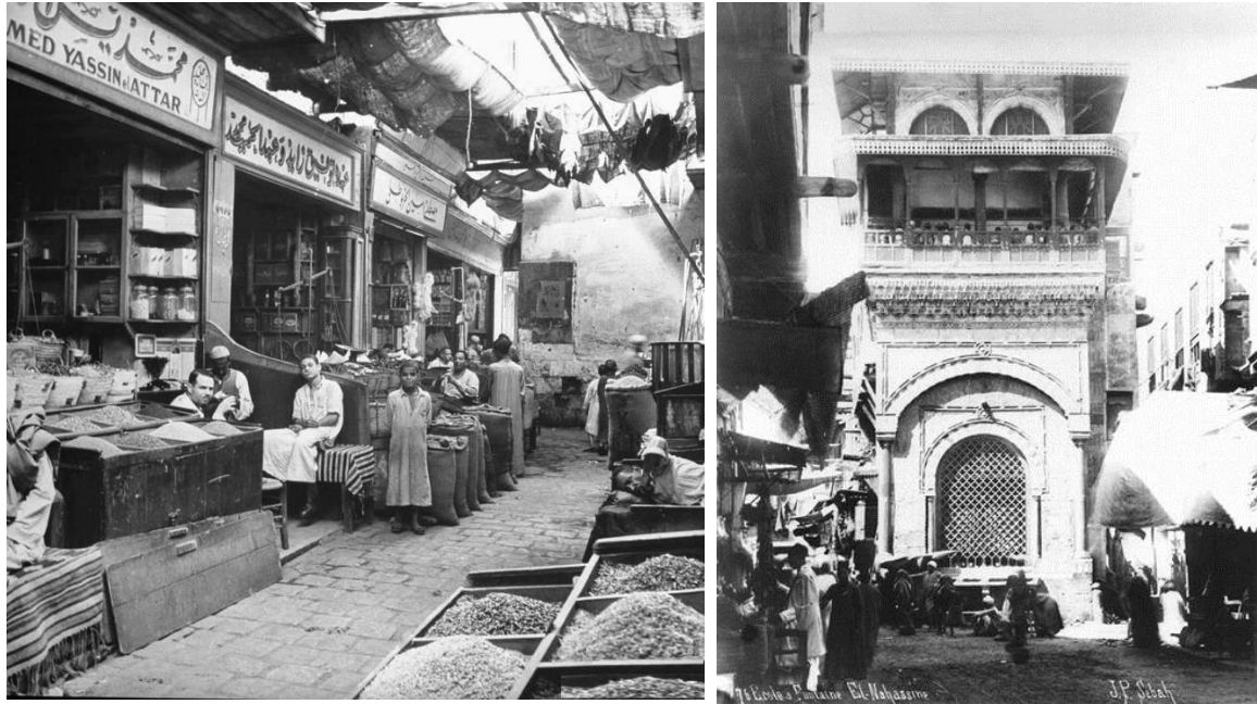
Figure 3-12 Old photos dated to the end of the 18th century for Al-Muizz Street show how people used their own techniques such as the movable tents to avoid direct solar radiation
