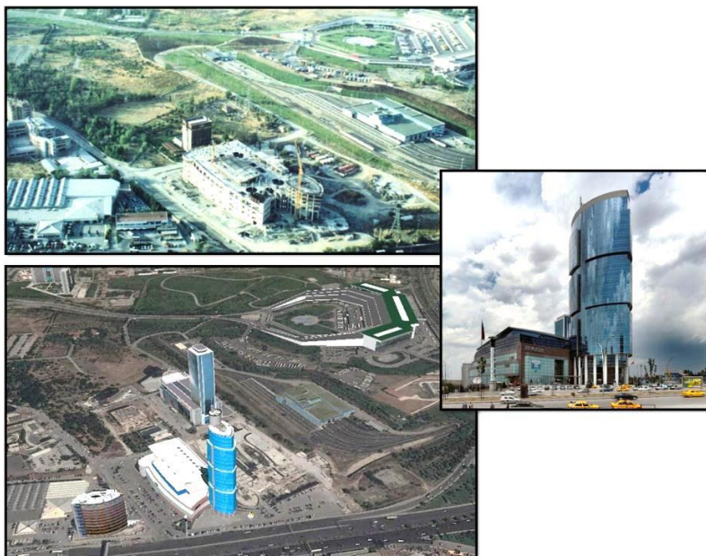
Figure 8.7. Armada Construction phase 1999-2002, Armada in use after 2002, Armada sky view of current phase and the construction of Armada-II project
