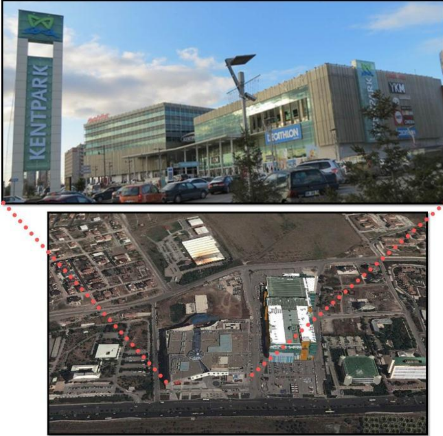
Figure 8.14. Kentpark Shopping Mall; aerial view together with Cepa Source: Author, 2011; Google Earth 2012
