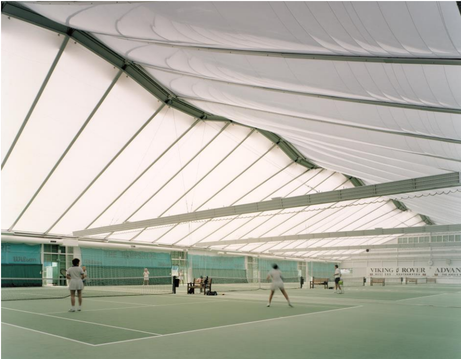
Figure 1-3: Eastleigh Tennis Centre, Southampton, UK
