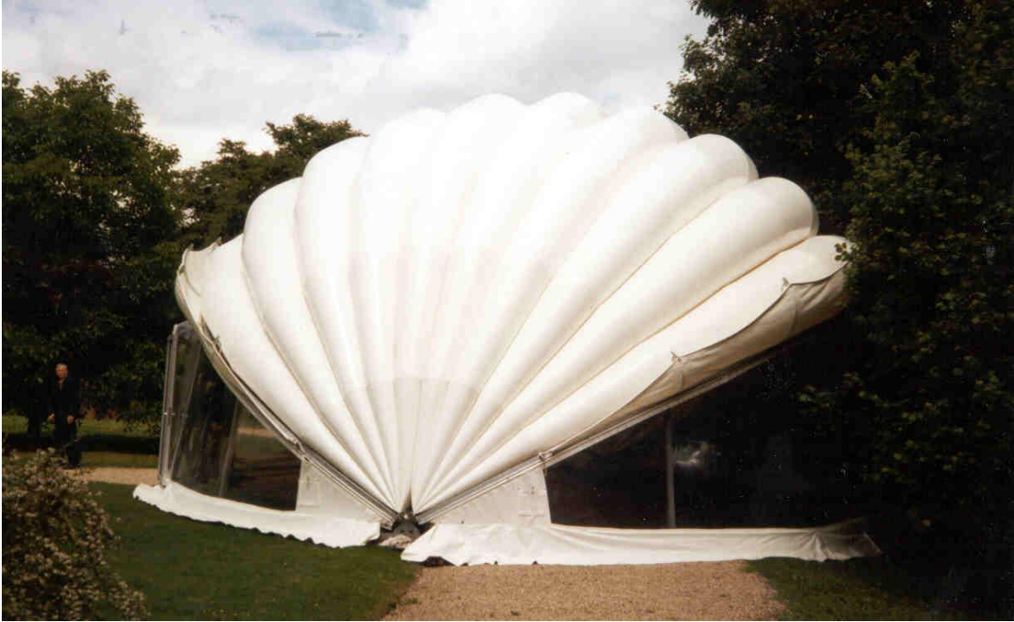
Figure 1-2: Tempory pneumatic structure
