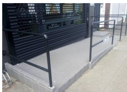
Figure 5-30 The ramp at H09
