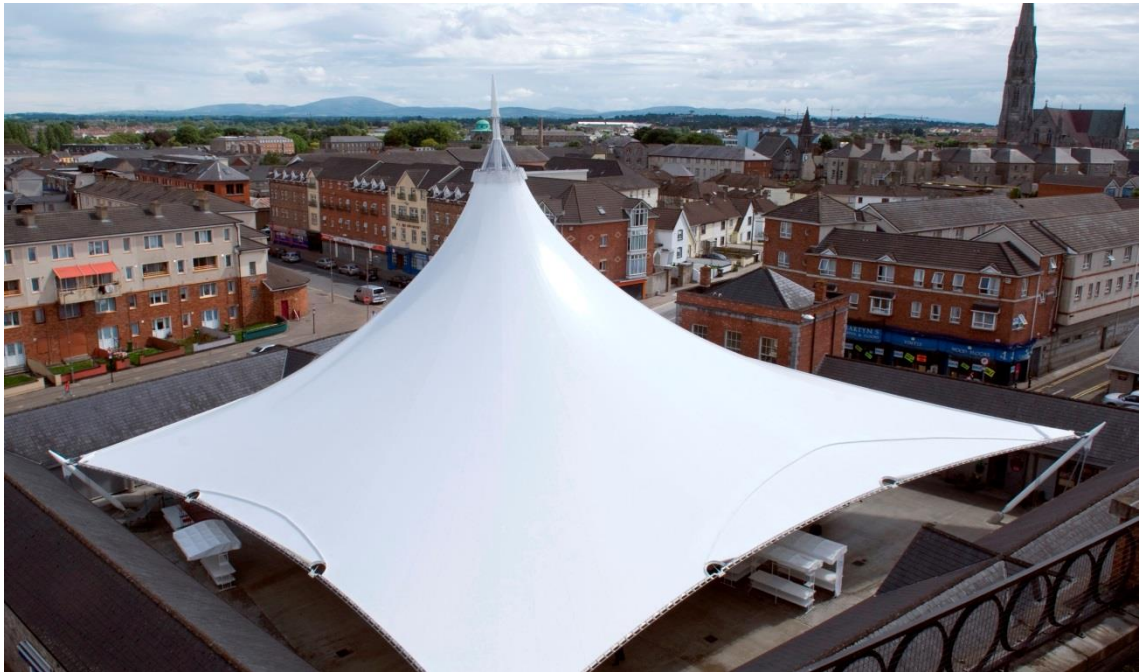
Figure 3.1 Milk Market, Limerick, a conic fabric structural form showing the anticlastic (doubly curved with opposite curvature in perpendicular directions) shape achieved by shearing the flat fabric panels during installation. © Schlaich Bergermann und Partner 2011
