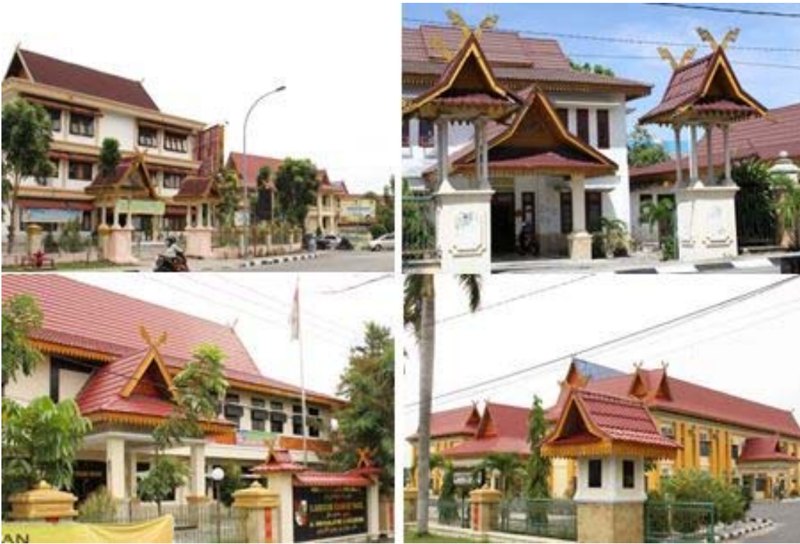
Figure 7.16 The Municipality Offices in Pekanbaru, 2012 The offices have been renovated or rebuilt between 2001-2010
