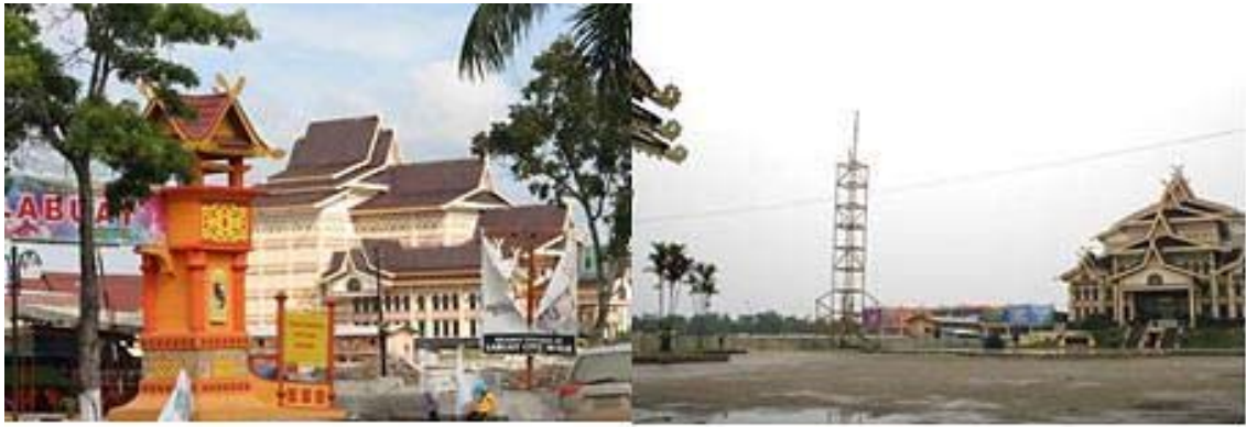
Figure 4.20 Demolishing Several Pavilions of Regency at Bandar Serai
