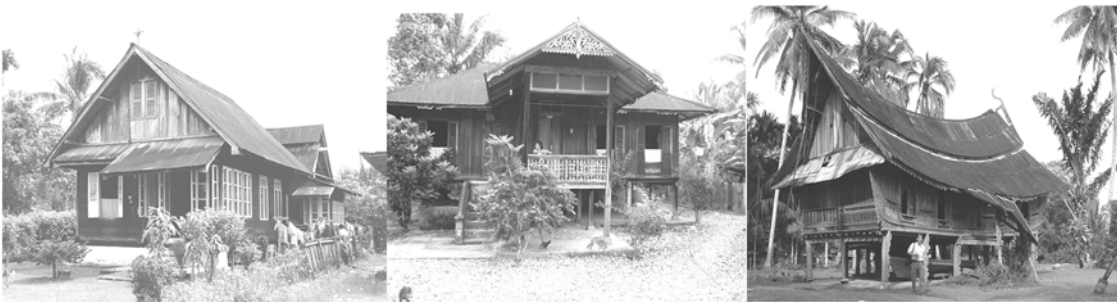
Figure 6.06 Basic forms of saddle roof on the east coast of Sumatera Left to Right: Belah Bubung , Limas , Lontik
