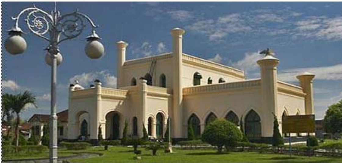
Figure 6.10 The Asseraiyah Hasyimiah Palace at Siak Sri Indrapura City
