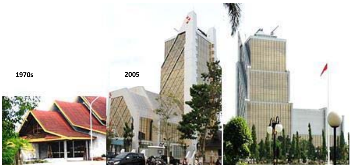
Figure 4.17 Dang Merdu: from Balai to Tower Building
