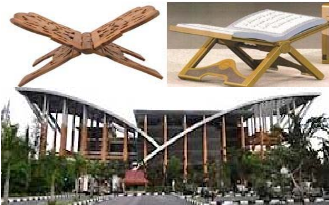
Figure 4.18 Soeman HS building, the Main Library of Pekanbaru, 2006
