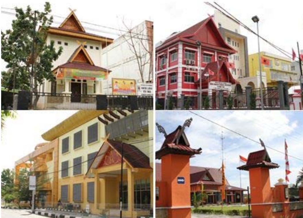
Figure 7.21 Dominant Colour on city buildings Yellow, green and red are most colours used on the buildings since 2001
