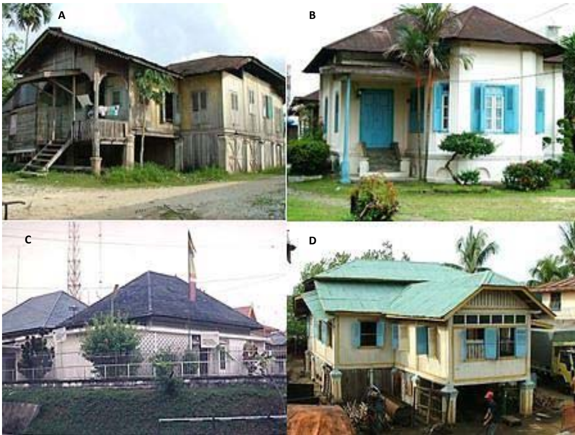
Figure 4.11 Traditional Houses at Senapelan A. Typical Stilts House; B the Dutch House; C House of Controleur ; D Rumah Singgah
