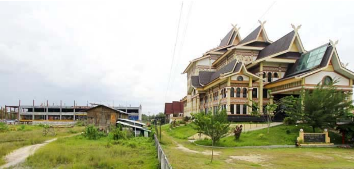
Figure 7.14 The construction of the Ritos Project has been neglected in Bandar Serai [left], 2014
