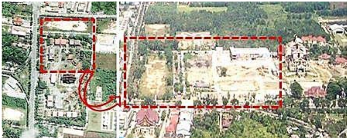
Figure 7.12 North-side of Bandar Serai compound has been demolished
