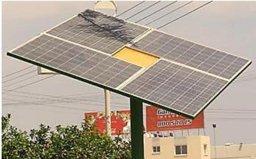
Figure C.13 PV with tracking system
