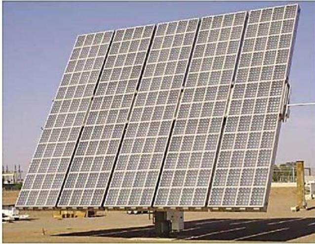
Stand-alone Photovoltaic system with tracking system and battery
