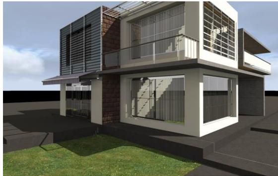
Figure 7.6 Solar collector integrated as shading
