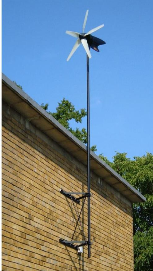
Figure C.15 Micro-Wind Turbine
