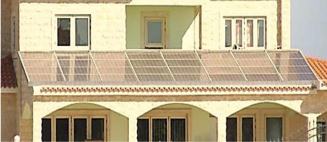
Figure C.10 Solar panels placed in a curtain wall type aluminium frame
