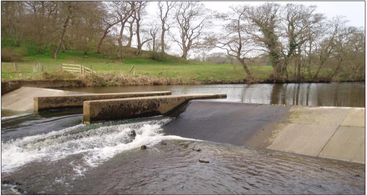
Figure 4.11 The structure of Mitford flow station (Ward, 2008).
