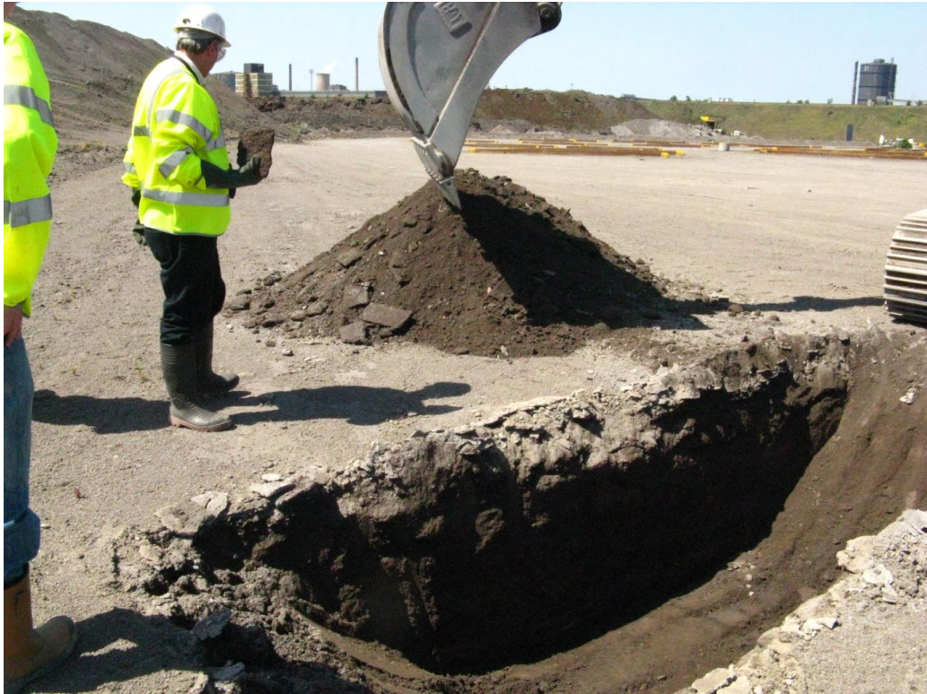
Figure C.1 – Excavation of YAR/TP3
