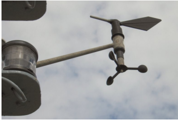
Figure 5.2: Anemometer and wind vane of the Bernicia
