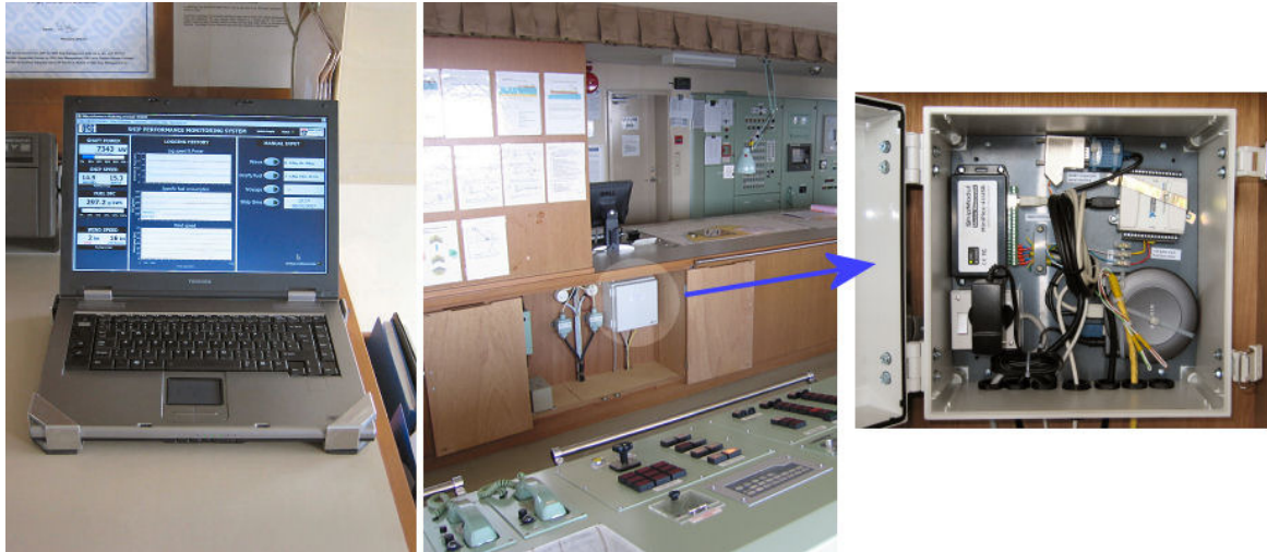
Figure C-1: Data acquisition system installed on the bridge of the Overseas Tanabe
