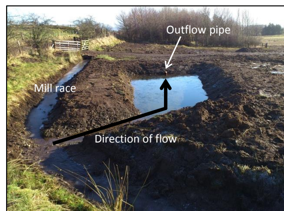
Plate 7.5: Single-cell RAF after construction (Feb 2012).
