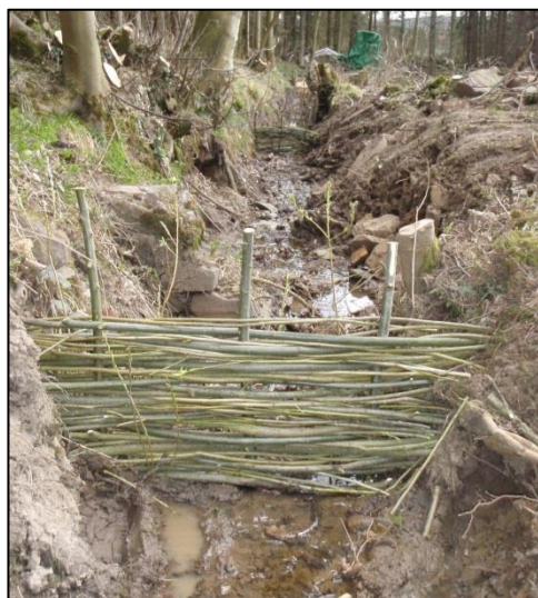
Plate 6.10: Woven willow dam after construction (taken 23/03/2011).
