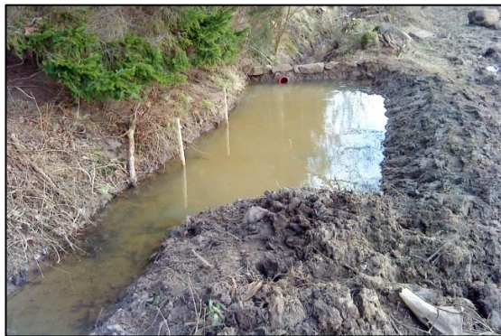
Plate 6.8: Sediment trap after construction.
