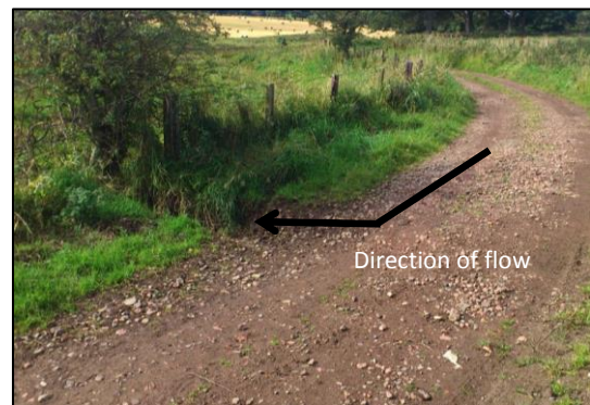
Plate 7.7: Inlet made to allow track runoff to enter single-cell RAF.
