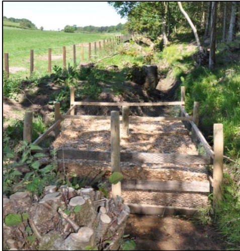
Plate 6.12: Fine filter feature containing circa 6 m 3 of wood chippings.
