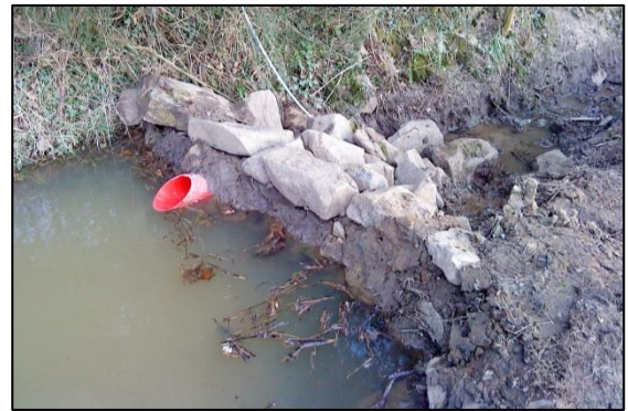
Plate 6.9: Rock and earth dam with outlet pipe.
