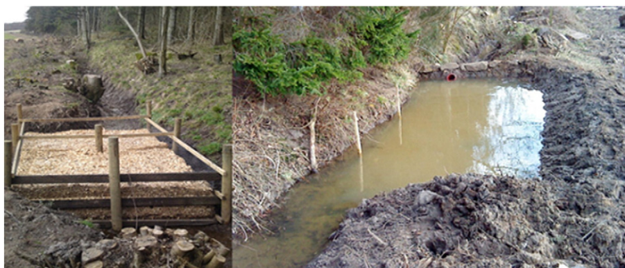
Fig. 6. Wood chip filter (left) and a sediment trap (right) placed in ditch upstream of RAF 12.
