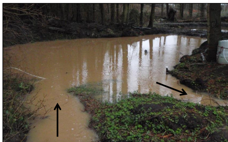
Plate 6.3: RAF 2 – sediment trap/online pond component during a storm event (sampled with auto-samplers – see data in 6.3.3). Black arrows indicate direction of flow.
