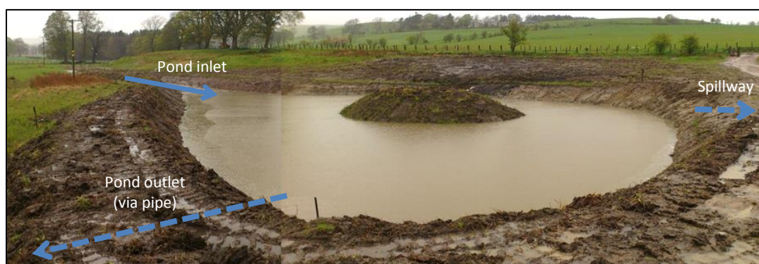
Plate 7.3: Main pond RAF after construction (Feb 2012).
