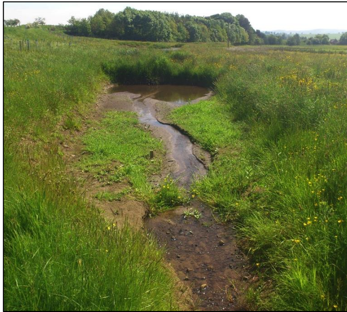
Plate 7.10: Cell one of the three-cell RAF contain 1 circa one year's worth of sediment (taken April 2013).
