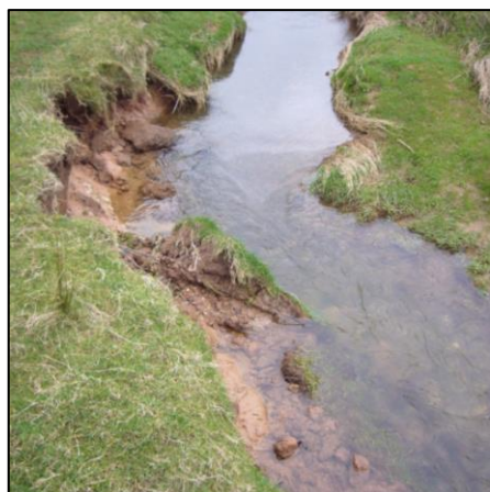
Plate 5.8: Bank collapse near Site 4, Sykeside Farm (February, 2011).
