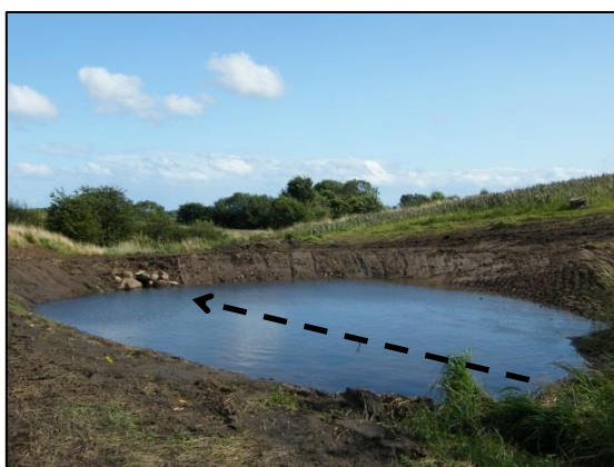
Plate 6.5: Online pond RAF after construction (September 2008).
