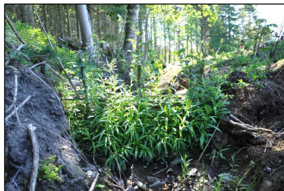
Plate 6.11: Living willow dam circa two months after construction (taken 02/06/2011).
