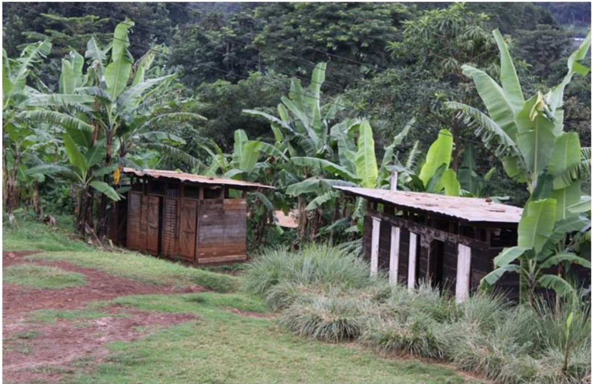
Figure 30: Typical pit latrines in a Hai village
