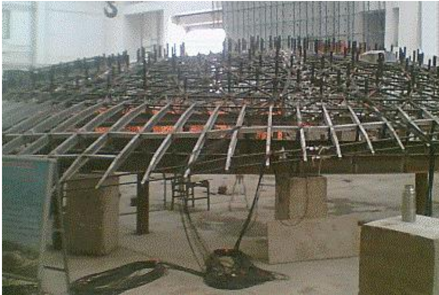
Figure 2-3: Illustration of roof monitoring through the use of strain gauge measurement (Yuan, 1991).
