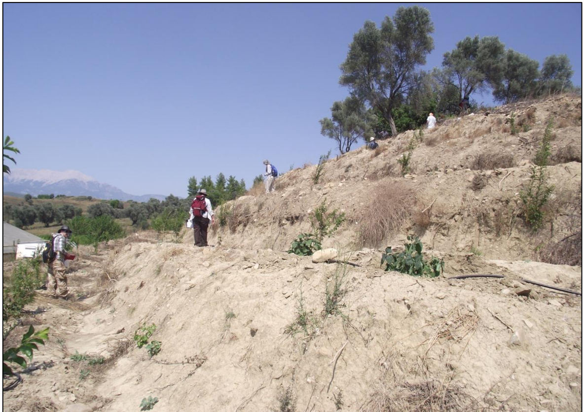
Figure 6.99: New bulldozed terraces in SU_10.
