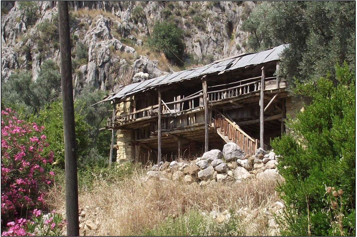
Figure 6.114: Ottoman timber and stone house in Kozan Köyü.
