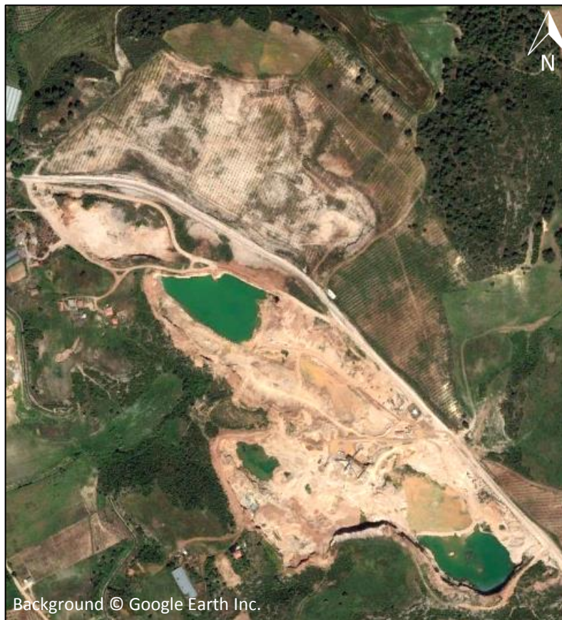
Figure 6.176: A quarry in 2011 after abandonment.
