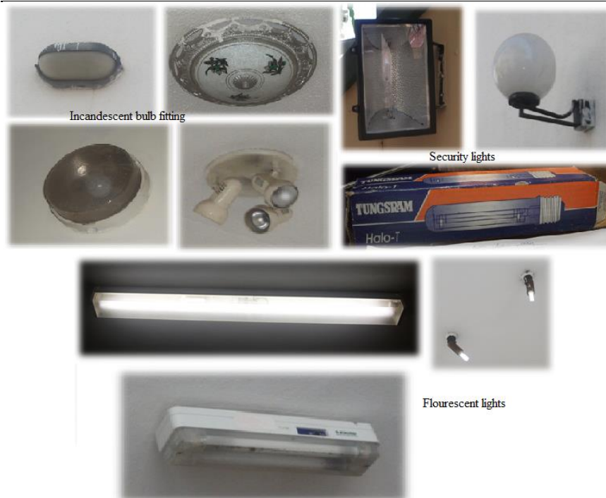
Figure 5-10 Lighting systems showing the range of available lighting from inefficient tungsten lamps to more efficient fluorescent lamps
