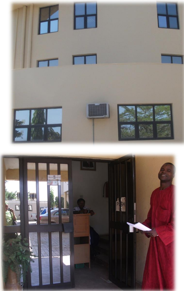
Figure 5-7 Single glazed, bronze tinted, aluminium framed windows and doors
