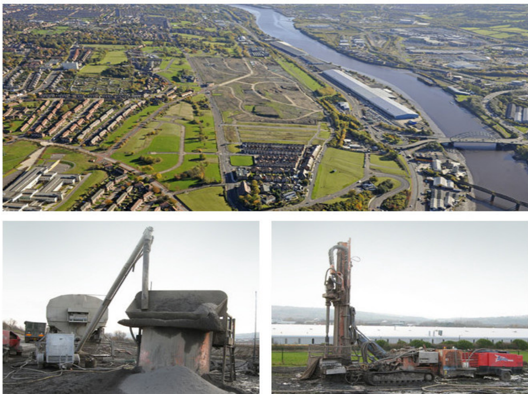
Figure 6.5 The preparation works in Scotswood Development area (source: www.GallyfordTry.co.uk )
