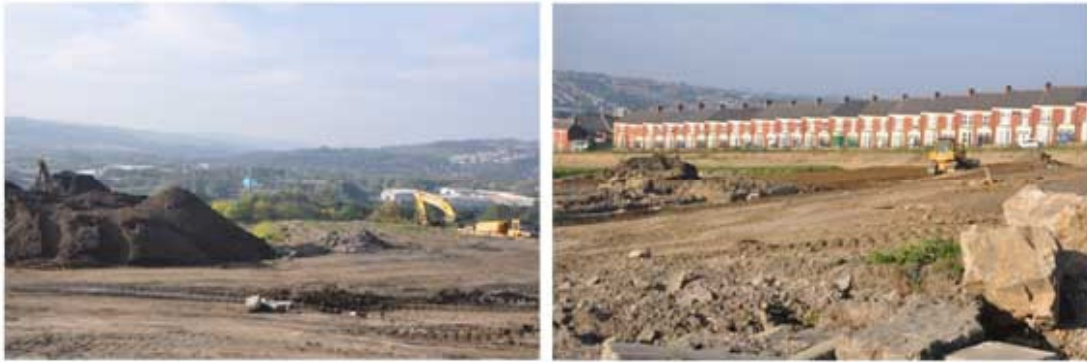
Figure 6.3 The redevelopment site under site preparation works (2011)
