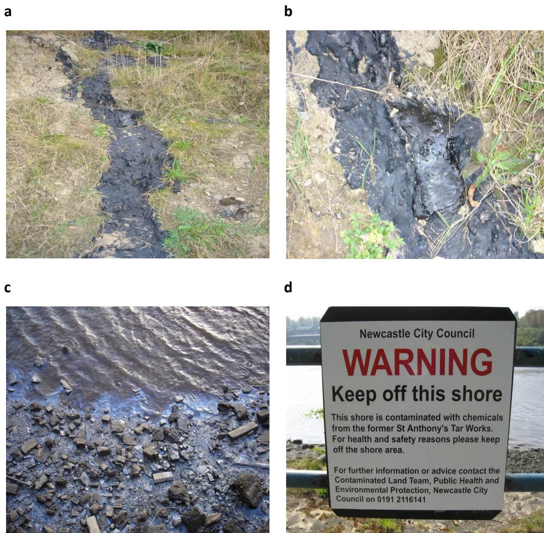
Figure 2-2: Evident pollution from St Anthony's Tar Works (photos taken by the author). (a) Solidified pitch permeating from soil. (b) Active pitch seepage from soil. (c) Seepage of hydrocarbons onto mudflats from quay wall into the River Tyne. (d) Public warning sign of contaminated land at the site.
