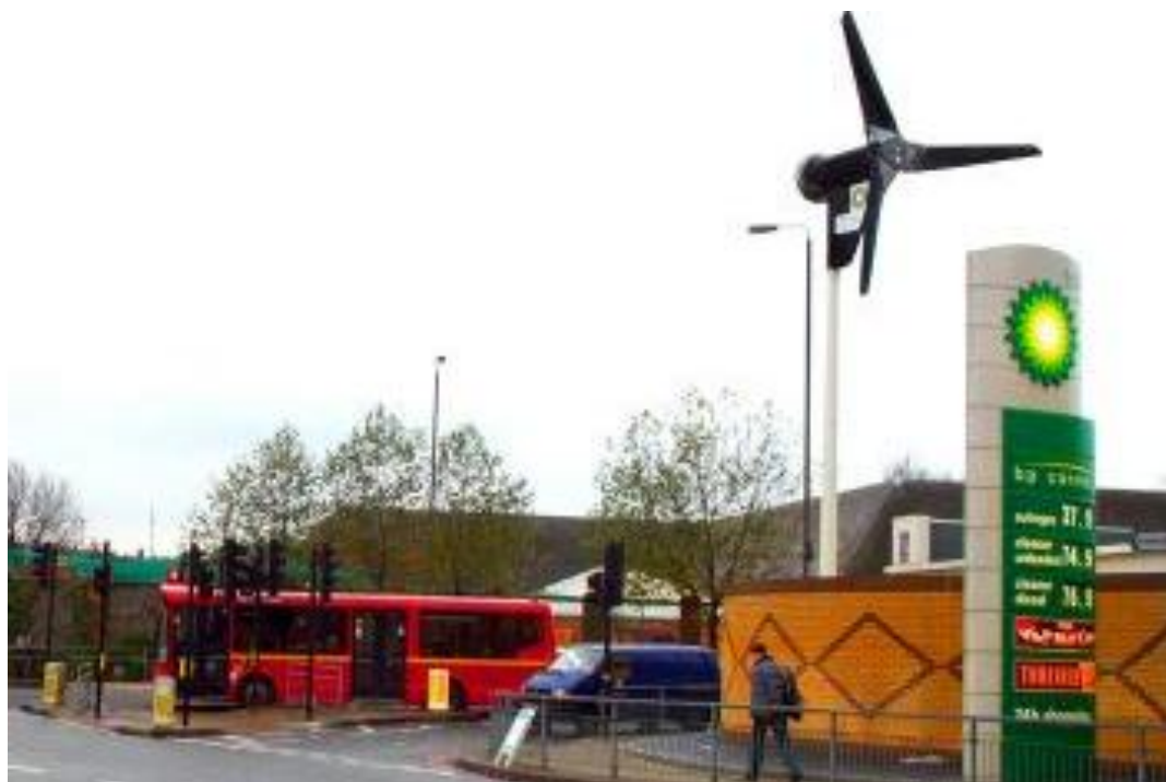
Figure 2.23 The building integrated wind turbine in a BP station in London (Stankovic et al. , 2009).
