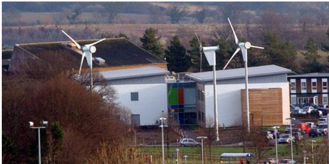
Figure 2.24 The three 15kw wind turbines at the ZEBRA project (Source: http://alnwick.journallive.co.uk/news/alnwick-divided-by-willowburn.html , accessed: 14/09/2012).
