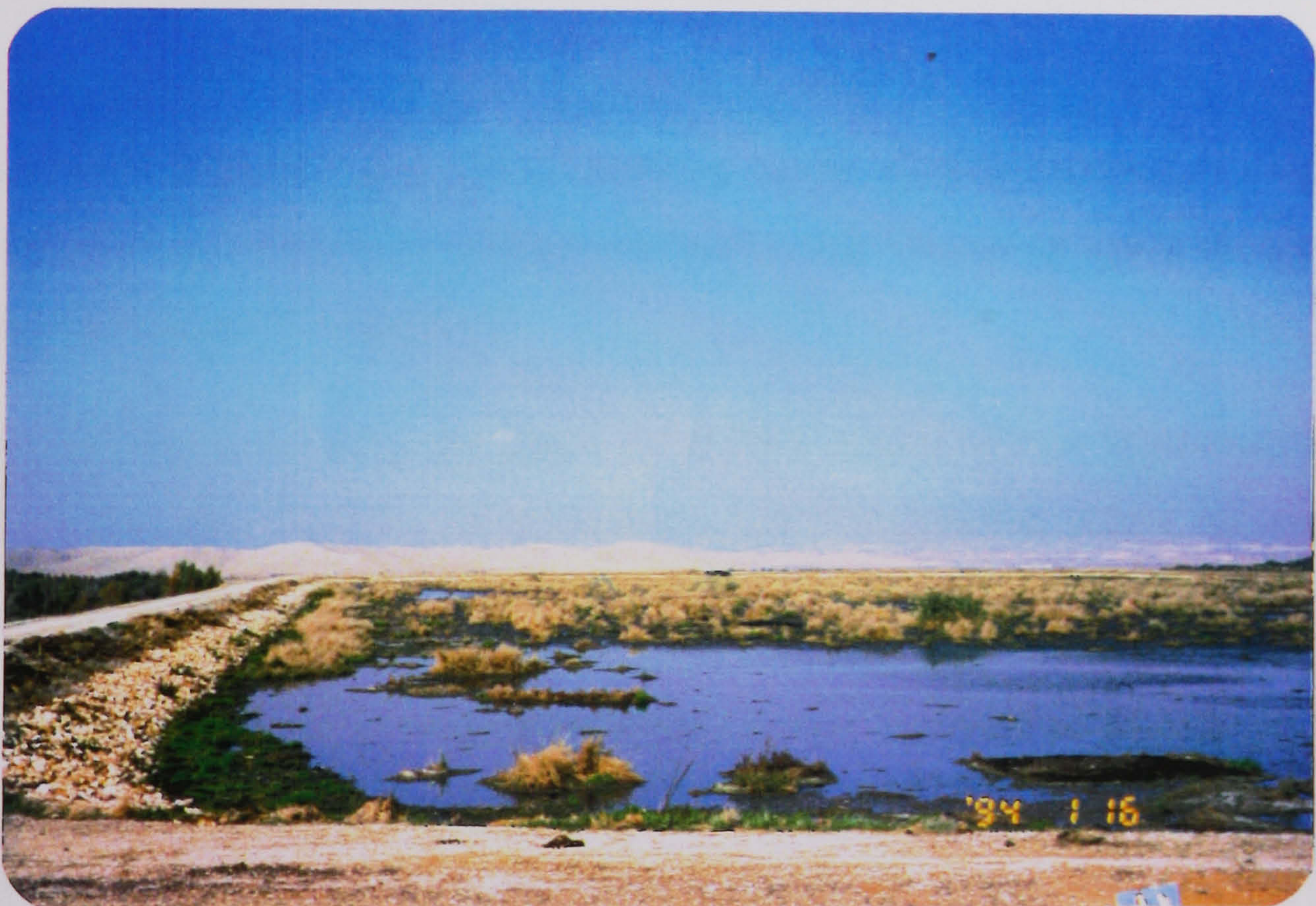
FIG. 6.5. Part of primary anaerobic ponds of Al-Samra WSP's system, showing the heavy floating scum on the surface of the pond
